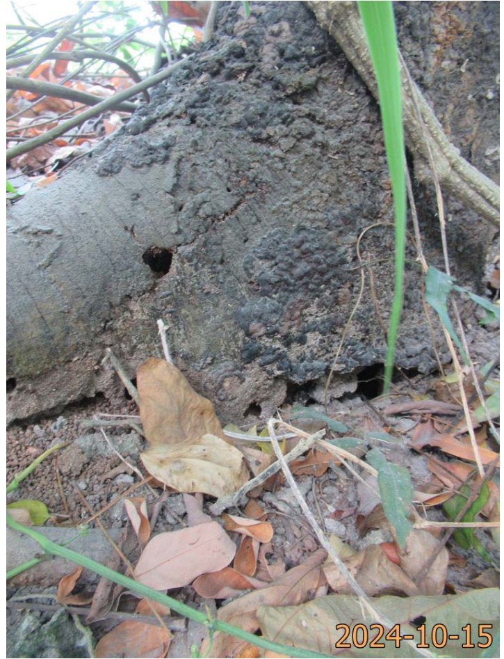
T15 Trace of termite
