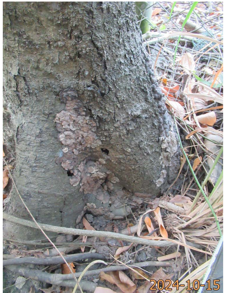
T16 Trace of termite
